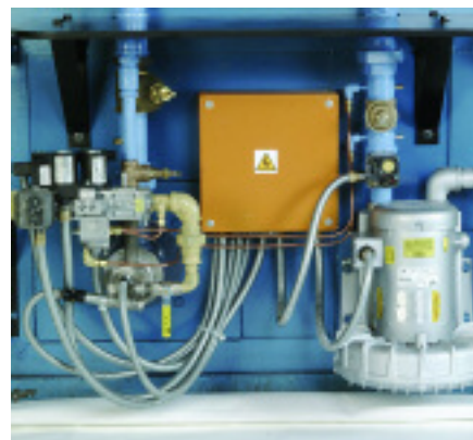
▲ General view of a typical Gas Burner.
